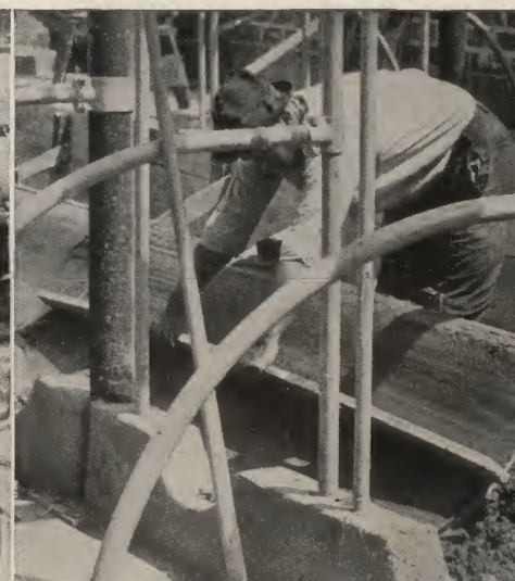
Forming curve with board and templets.
